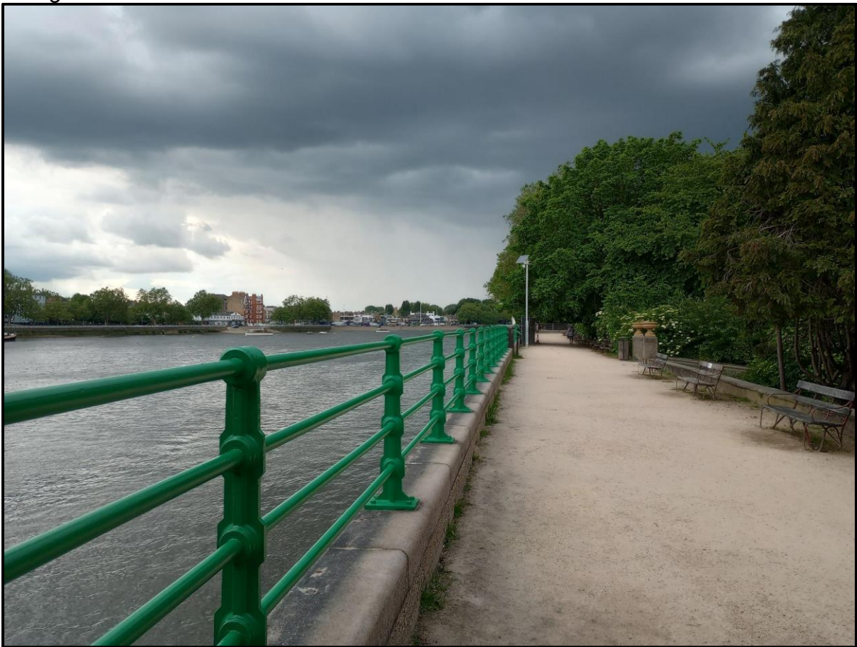
Refurbishment of 1km of riverside railings at Bishops Park, Spring 2024
